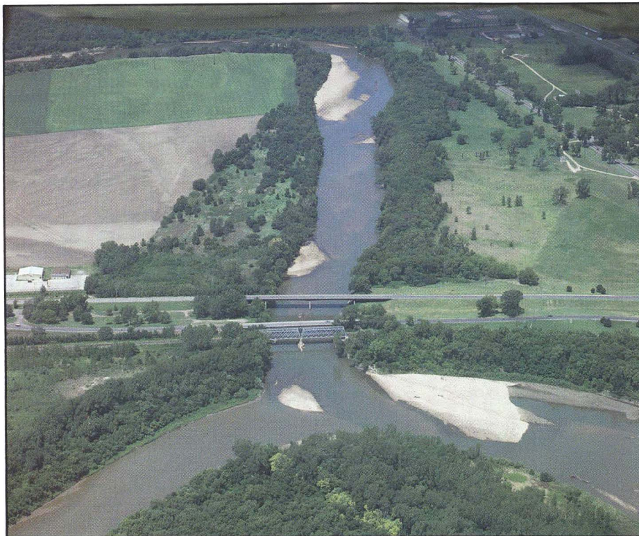
The clear waters of the Republican River below Milford Reservoir, at top, join the turbid, sediment-loaded waters of the Smoky Hill River, left, to form the Kansas River, right. More than 60 percent of the riverbanks between Abilene and Junction City have been cleared of woody vegetation. This has caused extensive bank erosion problems and hurt water quality downstream.
